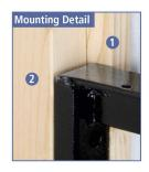
Concealed applications require ripping a 2" x 4" lengthwise, and mounting it (2) to the side of a standard 2" x 4" (1) stud.
