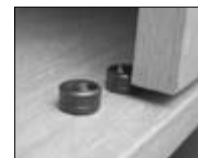
Screw Euro Door Stop at desired depth
